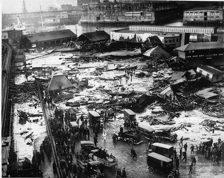
Figure 1. Aftermath of molasses tank failure
