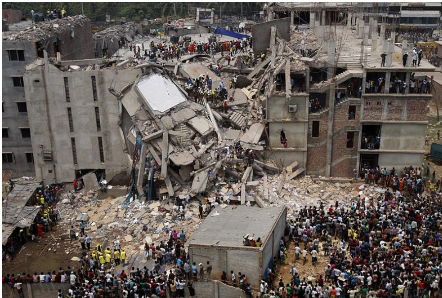
Figure 2. Aerial view of collapse.
